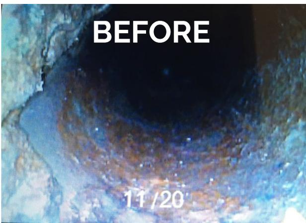
Before Altum's solution: hard fat fouling on the pipe's inner surface.
